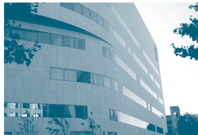
View of the McGovern Institute from Albany St.
